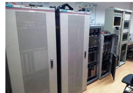
Linie BTS-BSC GSM/GPRS & NodeB-RNC 3G/UMTS– Siemens/NEC
