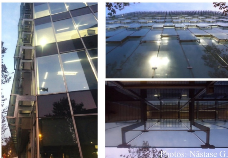
Figure 2. Side view, front view and under the cavity, Interface Building, Barcelona, Spain
