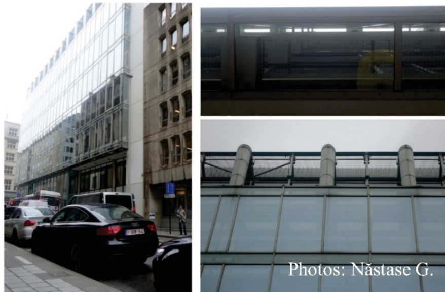
Figure 4. Double-skin façade on Brussimmo building, Brussels, Belgium
