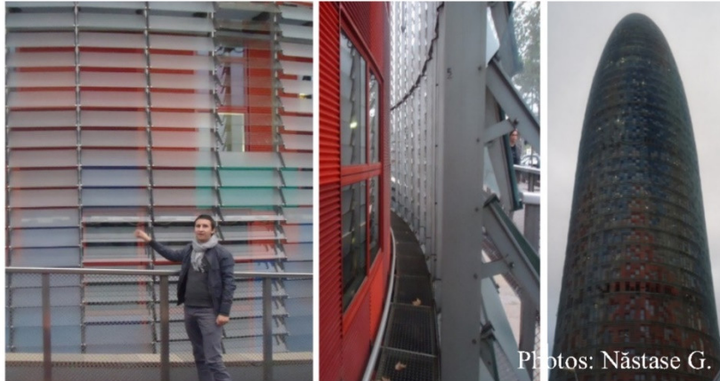
Figure 1. Exterior facade, the inner cavity and overview of Torre Agbar, Barcelona, Spain
