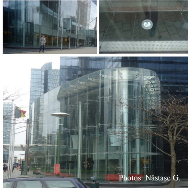
Figure 7. Detail and overall double-skin façade from North Galaxy Towers entrance, Brussels, Belgium
