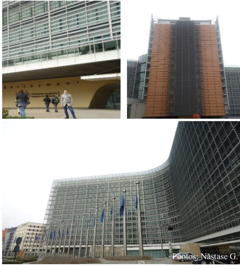
Figure 3. Front view, side view and overall view, Berlaymont Building, Brussels, Belgium
