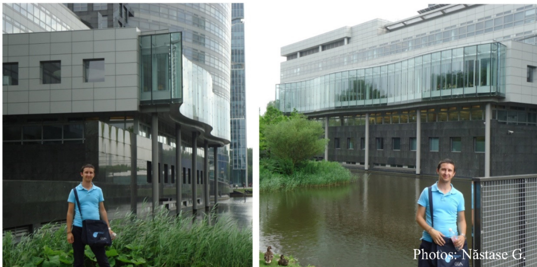
Figure 8. Views of double-skin façade, headquarters of ABN AMRO Bank, Amsterdam, Netherlands
