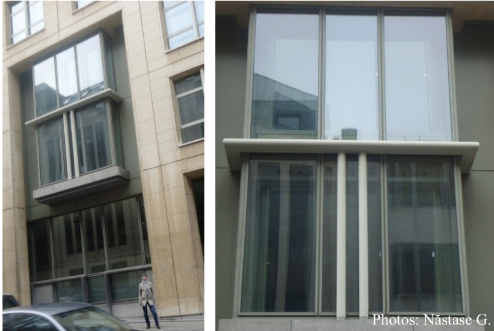
Figure 6. Double-skin façade, “box” type (southwest cardinal direction), DVV extension building, Brussels, Belgium
