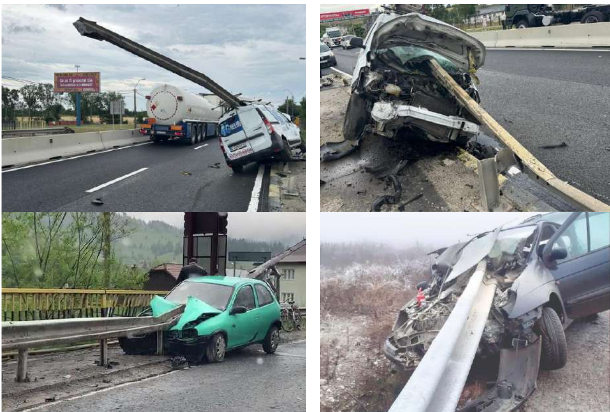
Fig. 2.9 Examples of collisions with safety barriers
