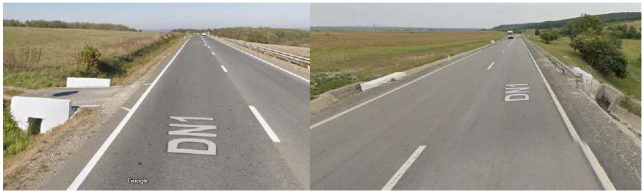
Fig. 2.6 Examples of hazardous drainage systems
