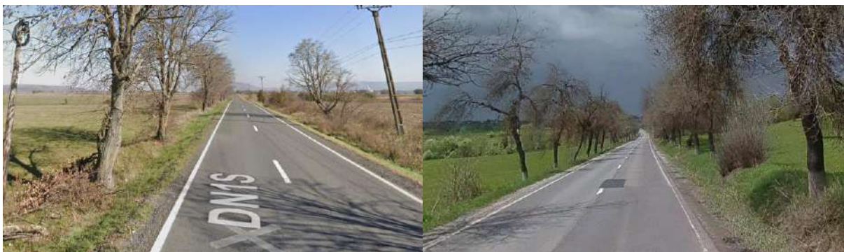
Fig. 2.1 Examples of hazardous trees located on the roadside
