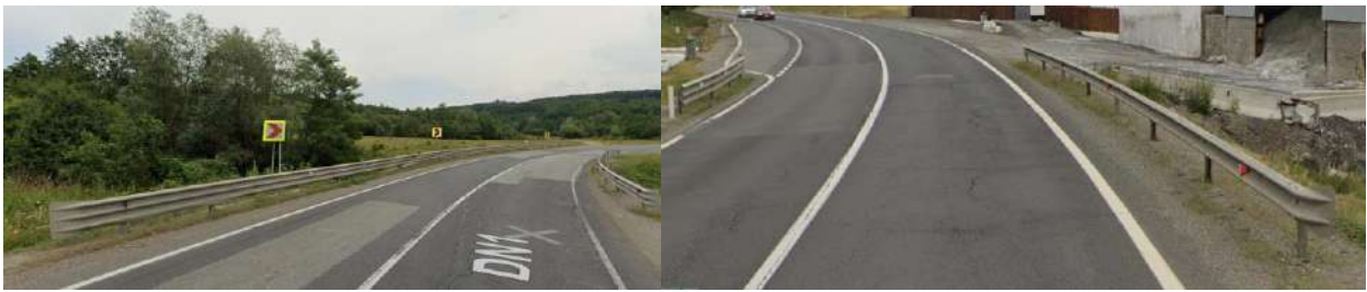
Fig. 2.10 Unprotected terminals
